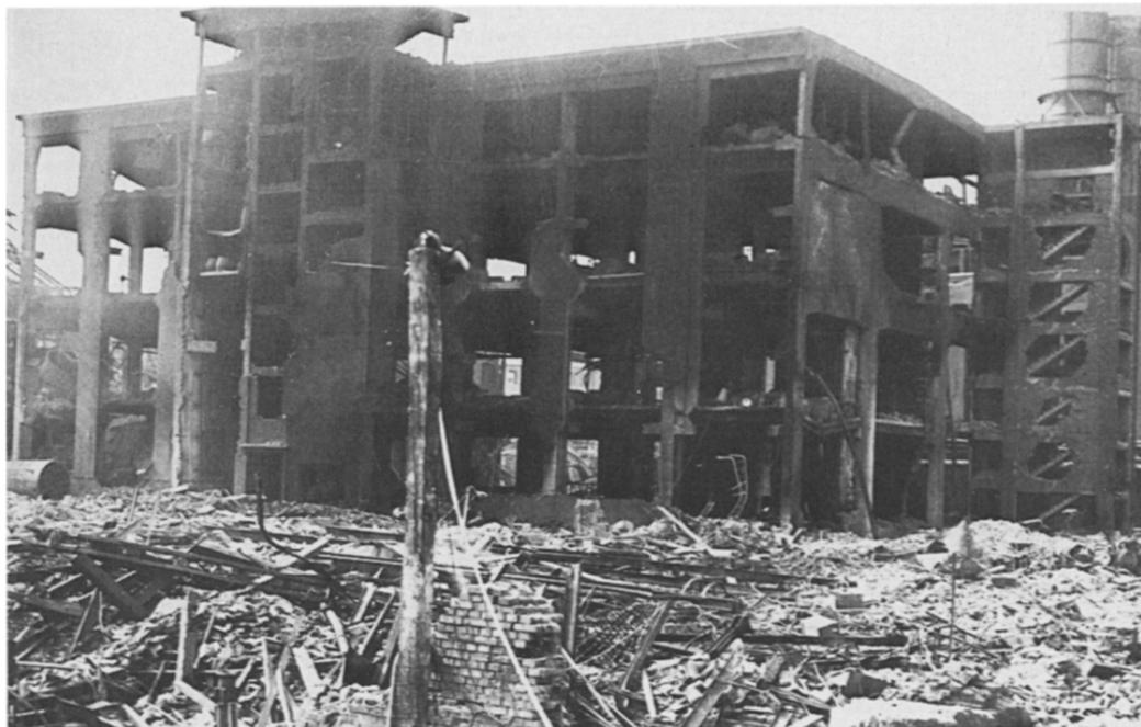
Fig. 7. Typical damage close to the 1948 vessel explosion at BASF (from [3]).
